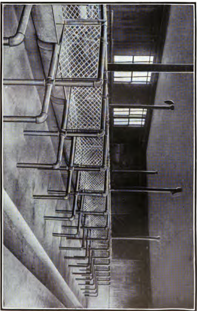
GAS PIPE STALLS, STEEL MANGERS AND CONCRETE FLOOR IN DAIRY BARN KENTUCKY AGRICULTURAL EXPERIMENT STATION
