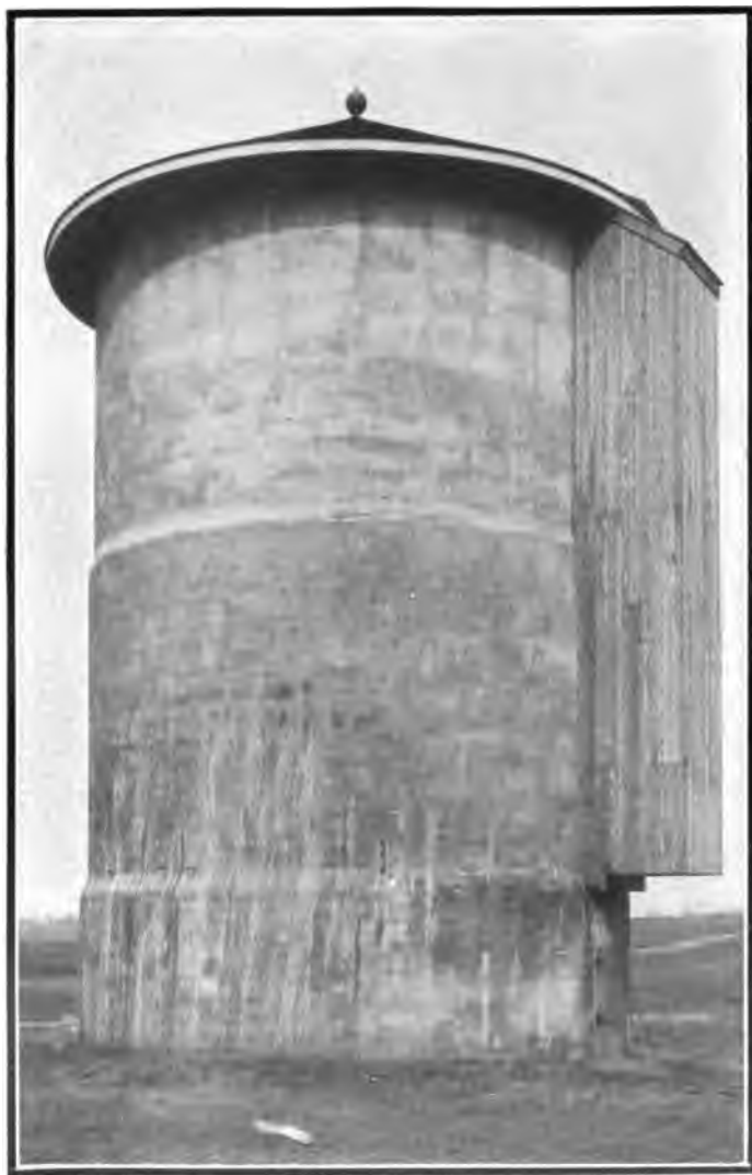
SILO OF SOLID CONCRETE WALLS
